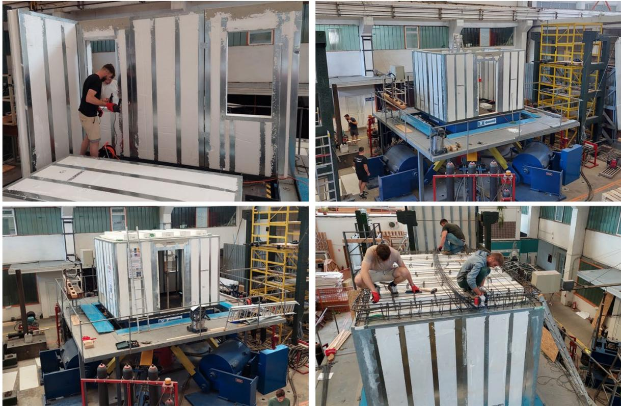
Fig. 7 – Assembly of THERMASTEEL panels and structure erection
