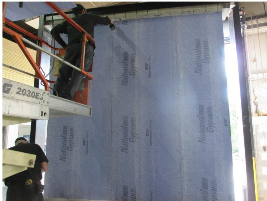
Photo No. 6 Installation of Exterior Type-X Gypsum
